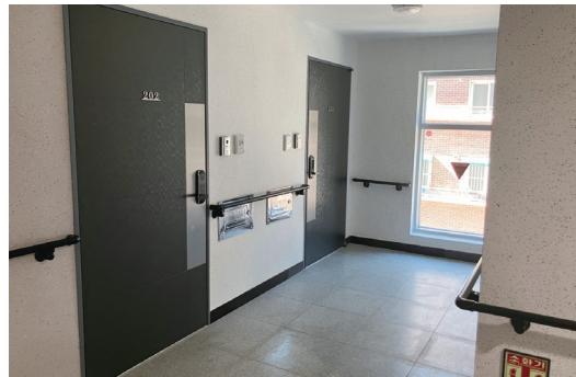
Corridor with safety bars (auxiliary handrails)
